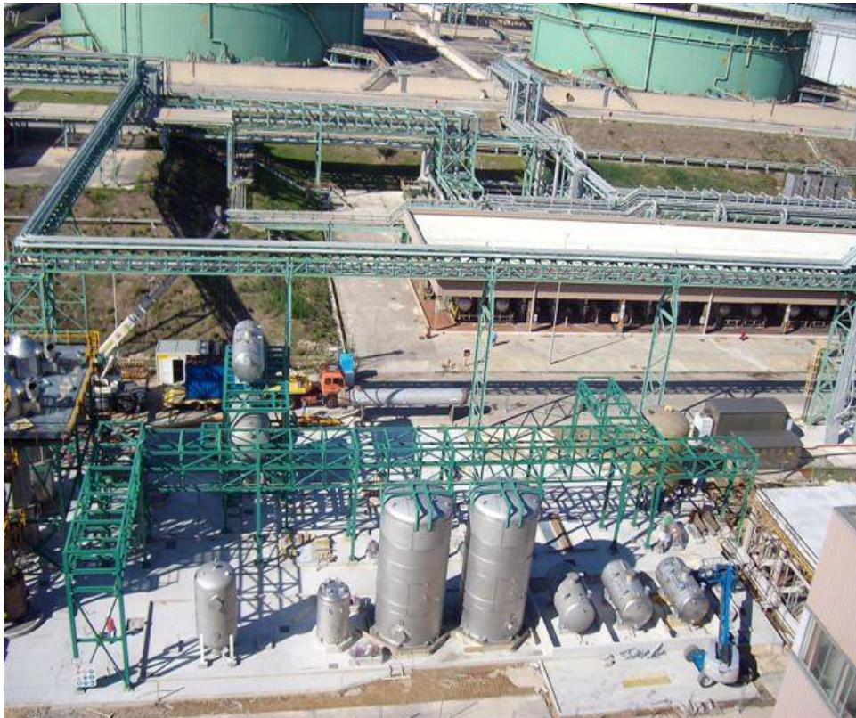
Work in progress at site - October 2009
